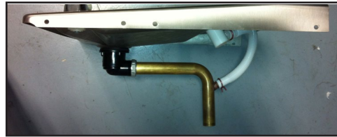
Exchange Drain hardware.
