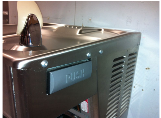
Fasten Basin Assembly in place.
