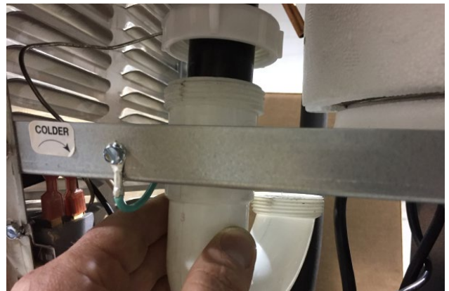
Reattach drain line to P-trap
